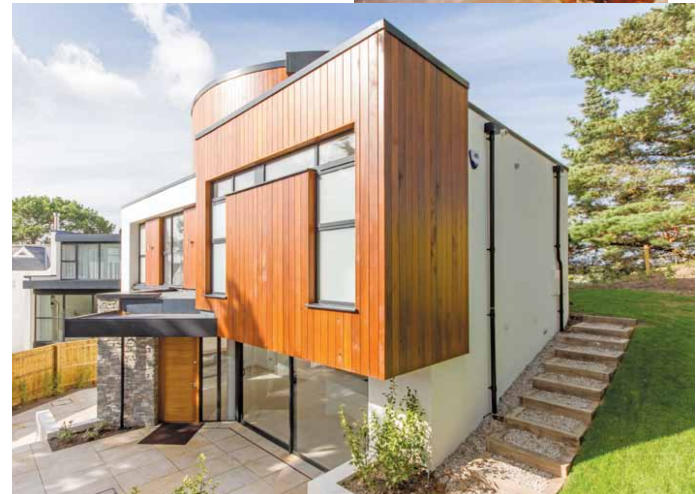
Ground conditions were the key challenge for this project in the prime location of Sandbanks, Dorset. The house sits on sand, which meant pile-driving foundations and insulated concrete formwork construction to ensure stability, according to owner and developer Neal Harvey of Bullform Developments (01962 858 810). Designed by David James Architects (01202 755 633; davidjamesarchitects.co.uk), with a build cost of around £3,229 per sqm, the four-bed house with views of Poole Harbour is for sale through Savills for £1.995million. (01202 708 888; savills.com)
